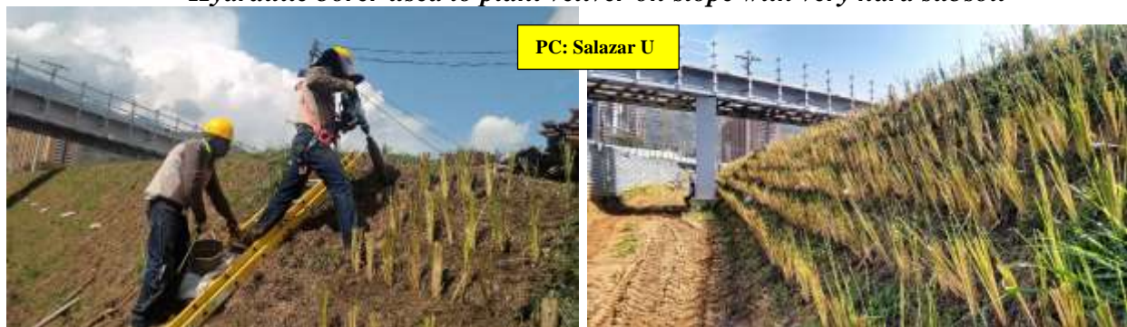
Hydraulic borer used to plant vetiver on slope with very hard subsoil
