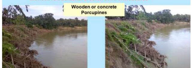
Ineffective traditional erosion control measures
