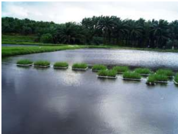
Vetiver pontoon treatment in industrial wastewater ponds in Malaysia (L) and China
