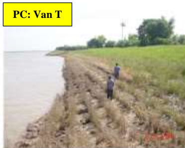
Three months after flooding showing dead vetiver
