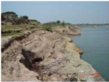
Erosion on the Mekong bank
