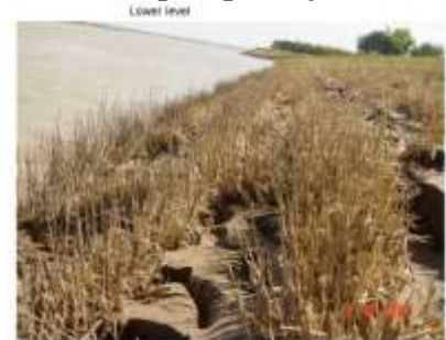
Dead vetiver on the deepest part of the bank
