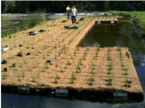
Vetiver pontoon treatment in industrial wastewater ponds in Australia
