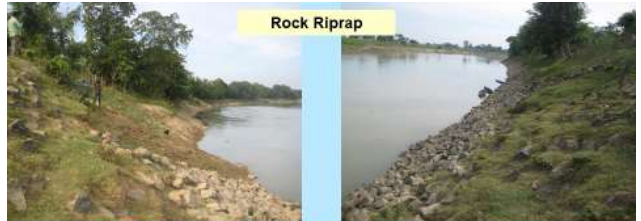
Ineffective traditional erosion control measures
