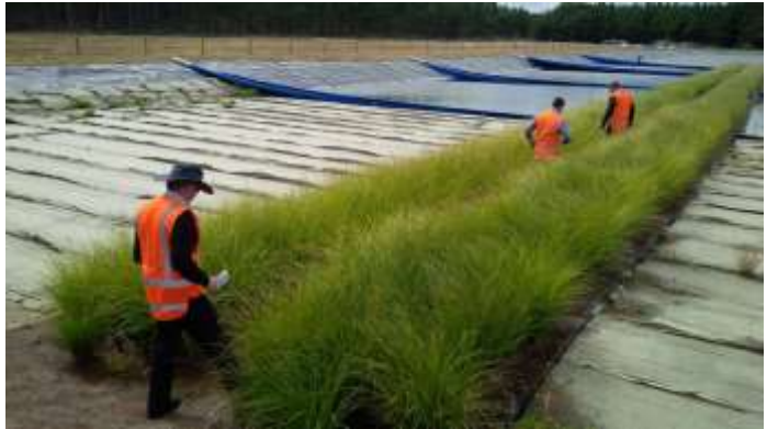
Vetiver pontoon treatment in industrial wastewater ponds in Australia
