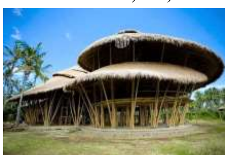
Vetiver roof and bamboo structure, Bali, Indonesia
