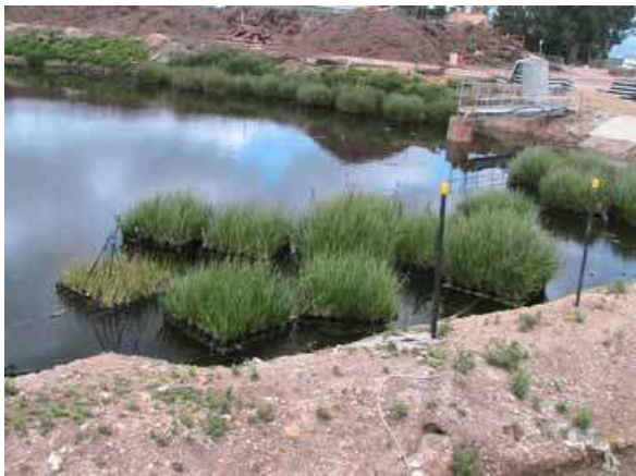
Vetiver pontoon treatment in industrial wastewater ponds in Malaysia (L) and China
